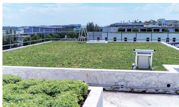
Images of The GEAR, Changi Business Park
