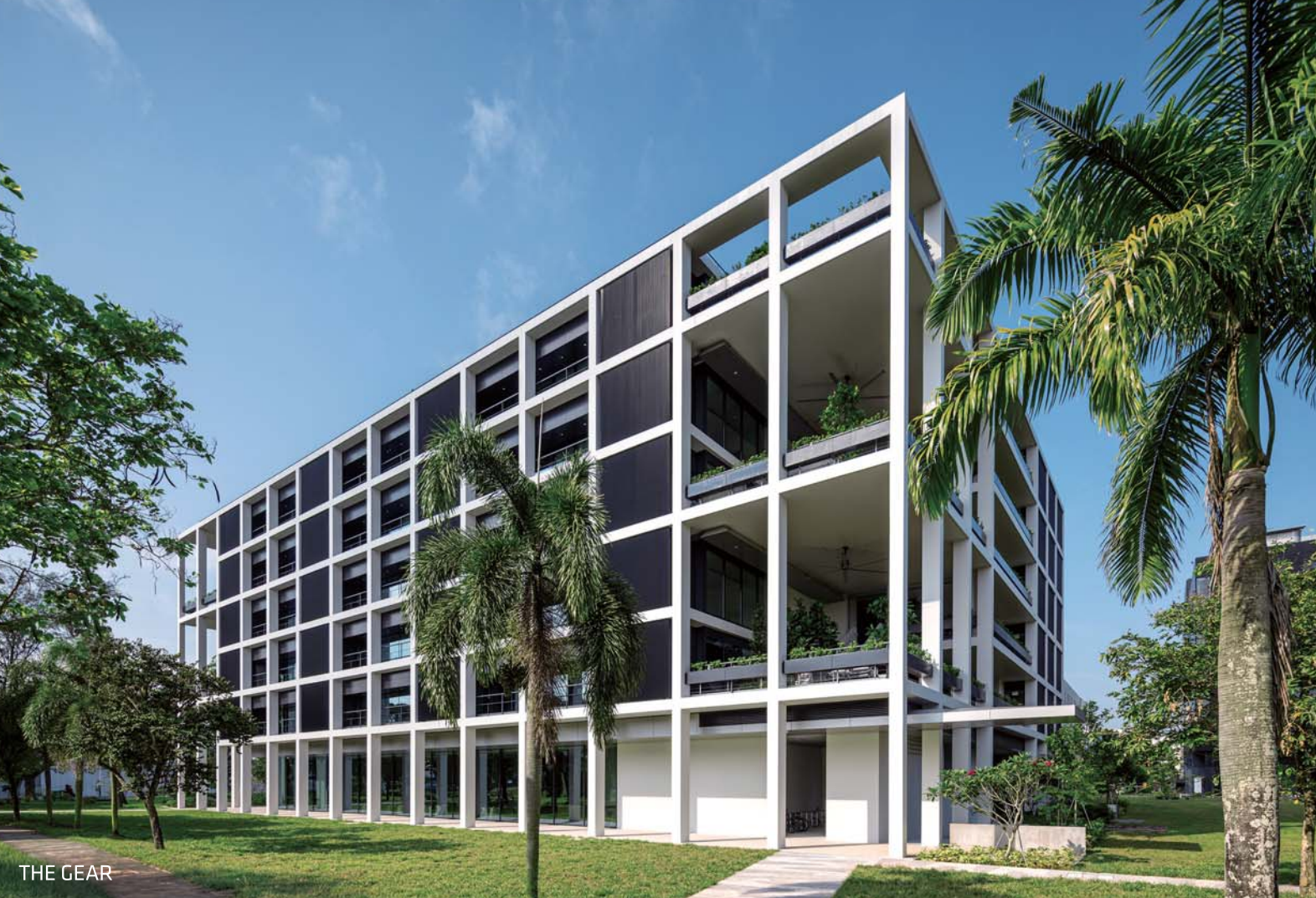
Images of THE GEAR, Changi Business Park
