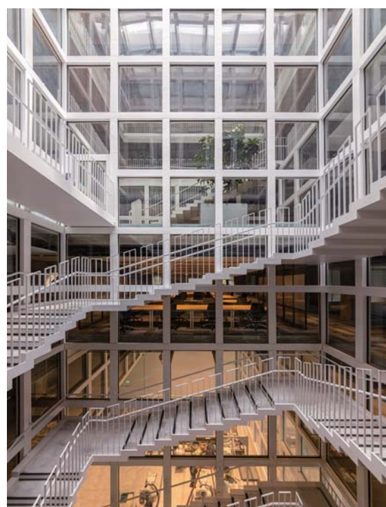
Images of The GEAR, Changi Business Park
