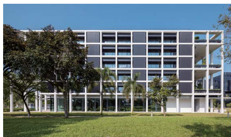
Images of The GEAR, Changi Business Park
